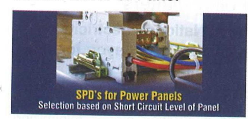
Surge Protective Devices are the most sensitive components in a power panel with response in nano seconds. The protective components such as MOV/ GD tubes Spark Gaps in SPD are always connected in parallel to the line.
