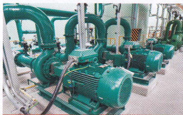
Impact of IEEE-650 Voltage Transient on Induction Motors Fed Through Ups and VVVF Starter
